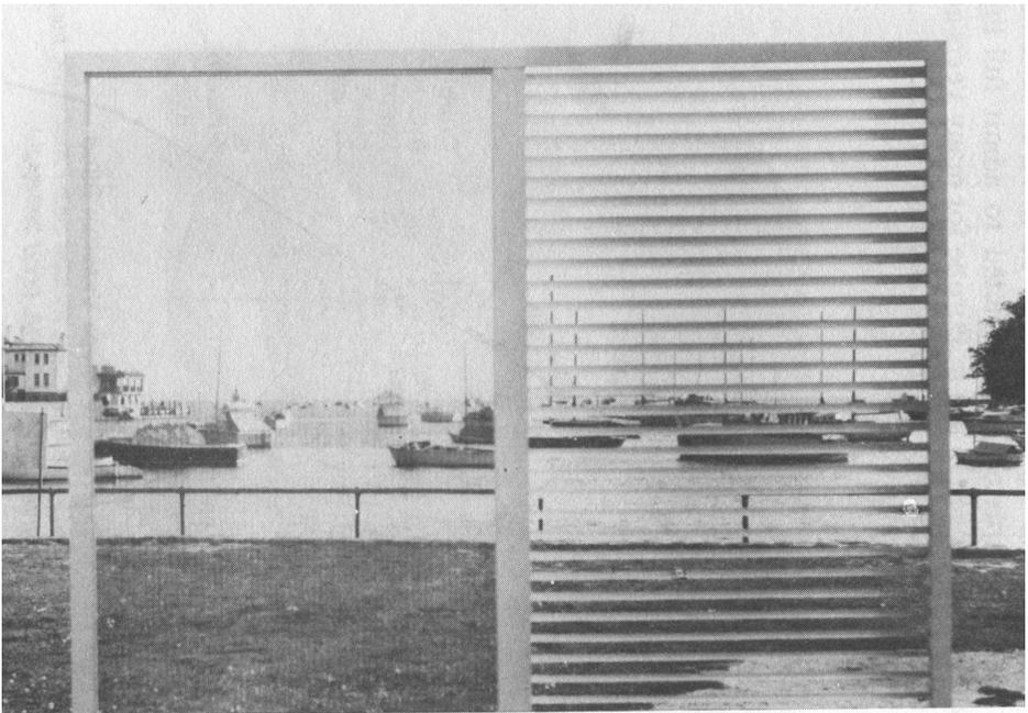
**Figure 6-26. Installation of Louvered Solar Screens**
