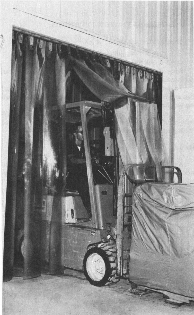
**Figure 6-4. Installation of Vinyl Strips on Forklift Door. (Photograph courtesy of MetalGlas Products, Inc.)**
