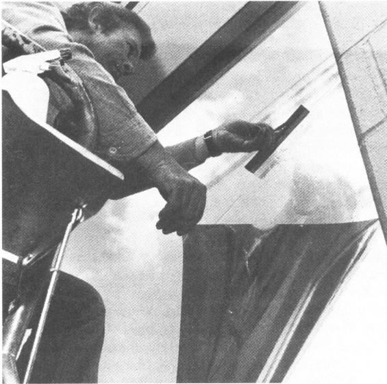
Figure 6-23. Application of Window Film. (Photograph courtesy of 3M Company)
