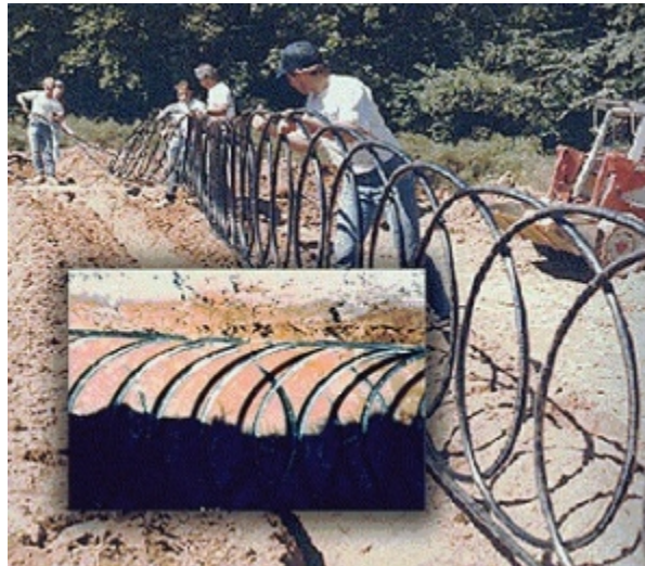
Upright slinky coil installation
