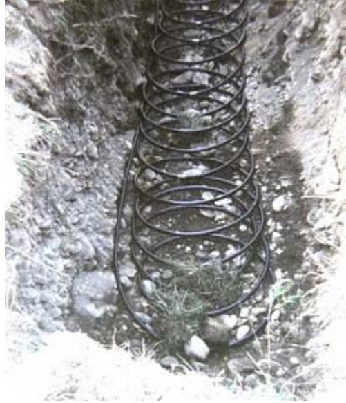
Upright slinky coil installation
